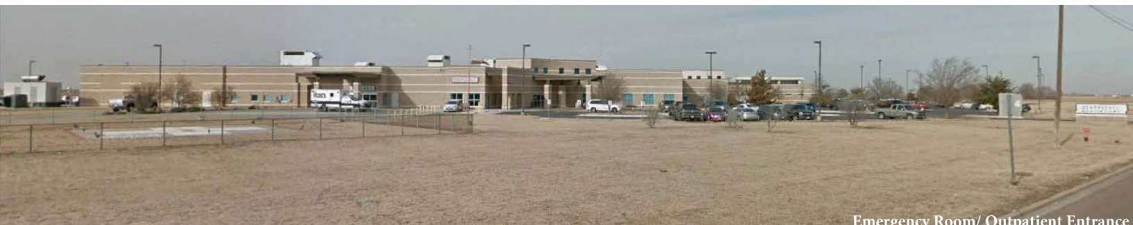
Emergency Room/ Outpatient Entrance
